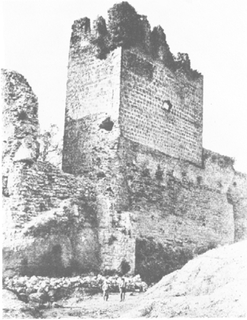
132. Trabzon, Citadel, Tower of John IV (Feature 16) from Southeast (1916), showing Classical Masonry A at Base, Darker 13th-century Masonry D3 with Ghost Crenellations, Courses of 14th-century Masonry E3, and Main Tower in Masonry F of 1458-60 (top lost between 1893-1916) above
